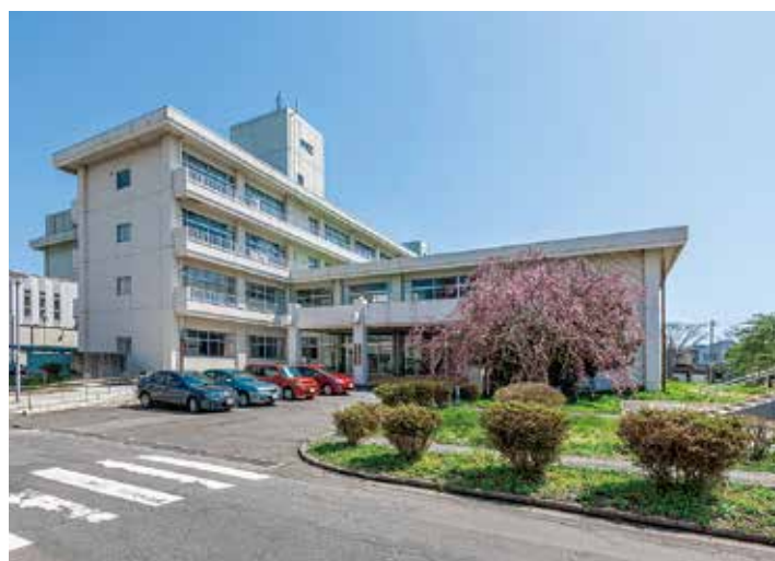
保健学科棟 Building for Health Science
