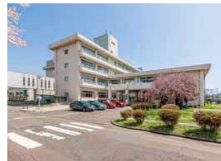
保健学科棟 Building for Health Sciences
