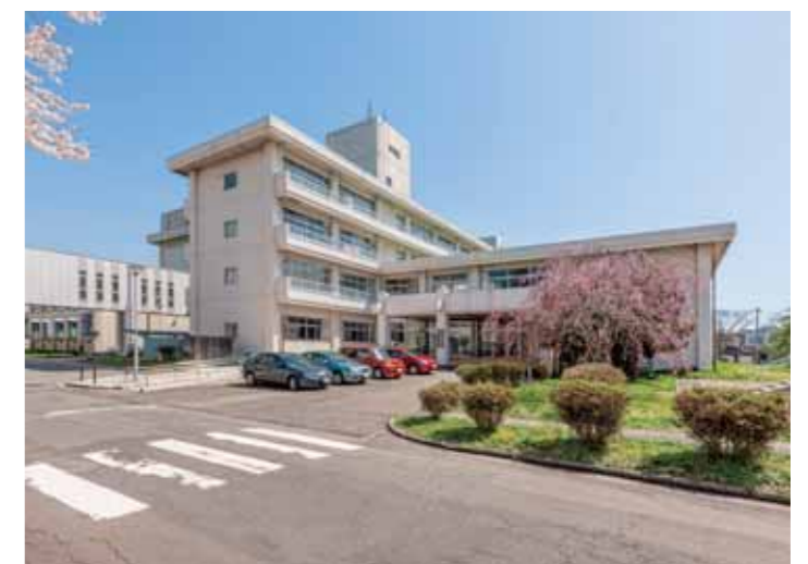
保健学科棟 Building for Health Sciences
