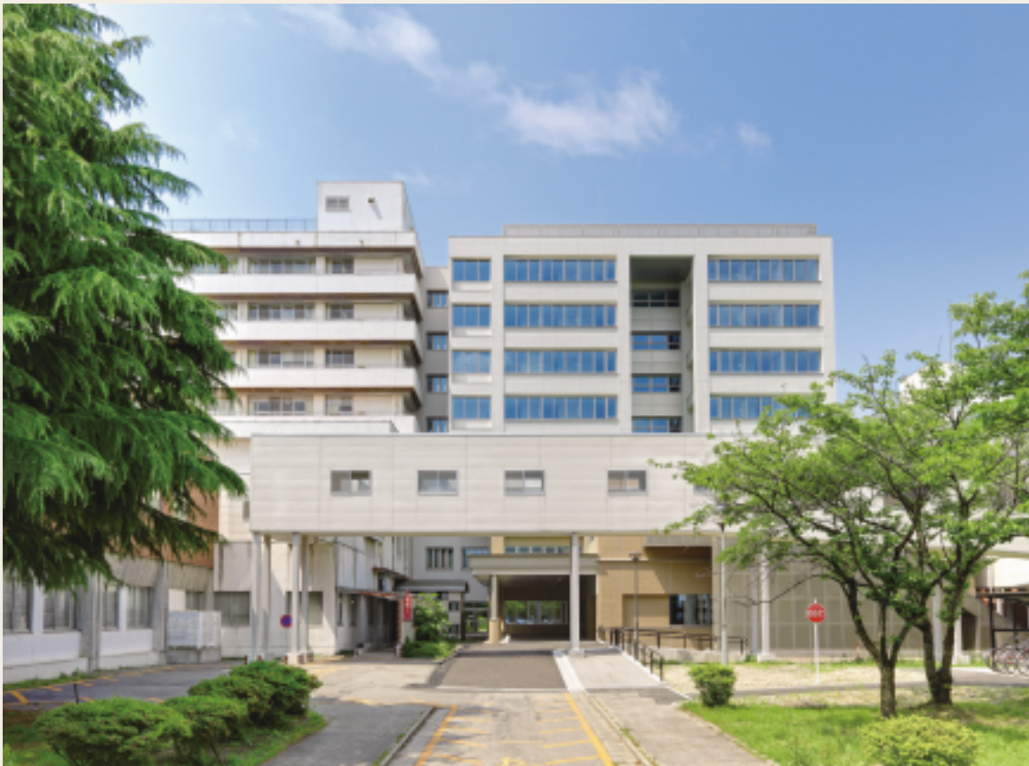
平成21年9月に開院予定の附属病院第二病棟 The New Wing of the University Hospital, due to open in September of 2009
